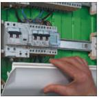
7 SIMPLIFIED ACCESS TO TERMINAL BLOCKS Chassis with removable, pivoting top and bottom parts for easy access to the terminal blocks
